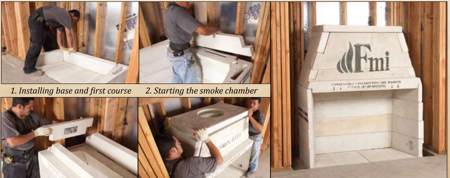
3. Easy to build smoke dome
