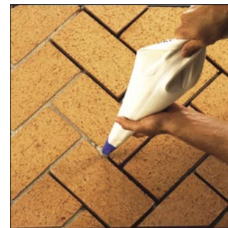
Fireplace grout lines are finished using the high temp, refractory mortar included.
